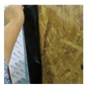
Remove 3" outside release paper and adhere DuPont™ Flashing Tape to the surface using firm hand pressure or a j-roller – be careful to avoid wrinkles and fish mouths.
