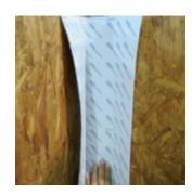
Working out from the corner, apply pressure and roll  $DuPont^{m}$  Flashing Tape outward to adhere product smoothly – be careful to avoid wrinkles and fish mouths.
