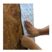
Remove the remaining 6" release paper and apply the DuPont<sup>TM</sup> Flashing Tape to the surface using firm hand pressure or a j-roller. Adhere product smoothly – be careful to avoid wrinkles and fish mouths.
