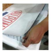
Fold DuPont™ Flashing Tape in half lengthwise, along split between two release papers and apply pressure to the fold to create a sharp crease.
