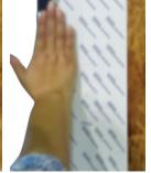
Remove 3" outside release paper and adhere DuPont™ Flashing Tape to the surface using firm hand pressure or a j-roller. Adhere product smoothly – be careful to avoid wrinkles and fish mouths.
