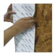
Working out from the corner, use firm hand pressure or a j-roller to roll the DuPont™ Flashing Tape outward. Adhere product smoothly – be careful to avoid wrinkles and fish mouths.
