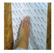
Remove the remaining 6" release paper and apply the DuPont™ Flashing Tape to the surface using firm hand pressure or a j-roller.
