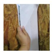
Starting at the bottom of the wall, place the fold flush against the inside corner with the perforated release papers facing out.
