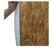
Starting at the bottom of the wall, align the folded edge with the corner so the perforated release papers are facing out.
