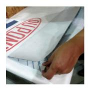
Fold DuPont™ Flashing Tape in half lengthwise, along split between two release papers and apply pressure to the fold to create a sharp crease.
